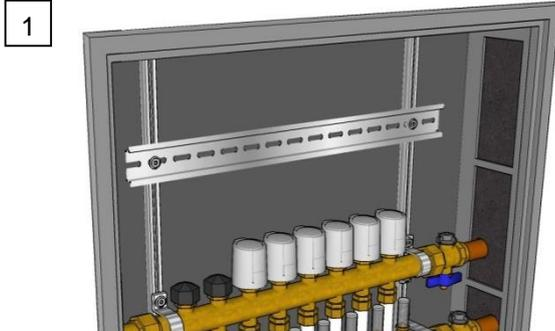
1 Install a DIN rail on-surface or in the heating circuit distributor cabinet, or use an existing one.
